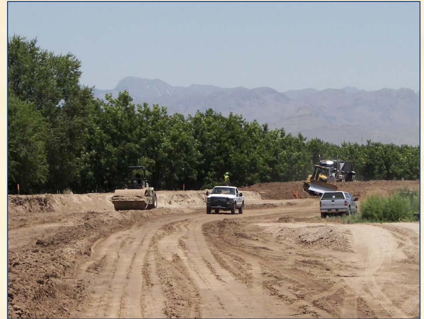
Levee rehabilitation near Vado, NM
