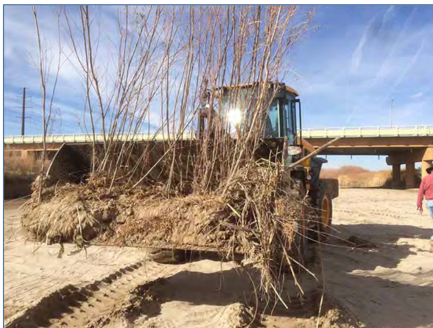
Removing coyote willows for transplanting at Anapra Bridge, February 2018
