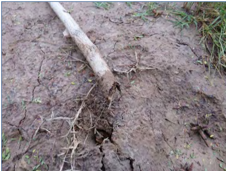
Example of cottonwood that rotted at the base at Anapra Bridge, 17 October 2018
