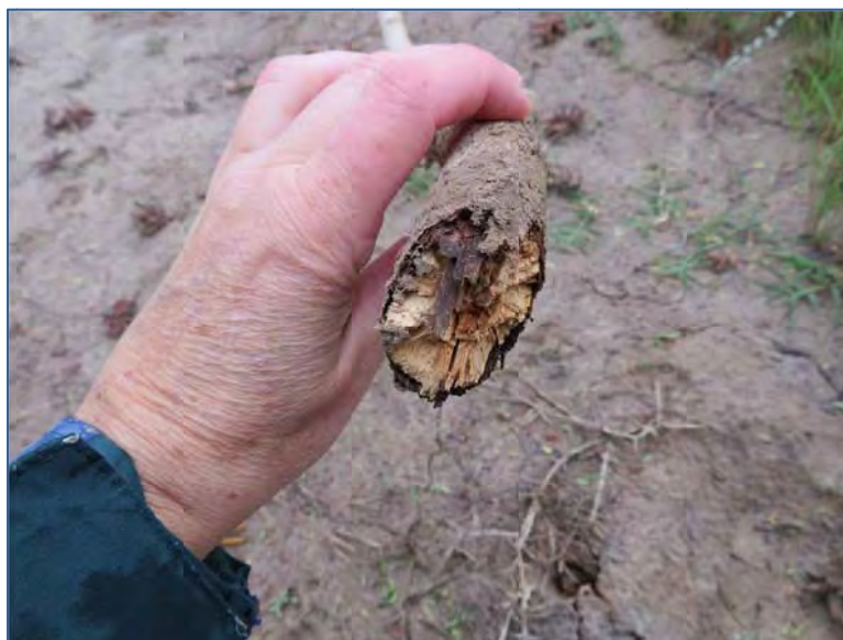
Base of rotted cottonwood at Anapra Bridge, 17 October 2018
