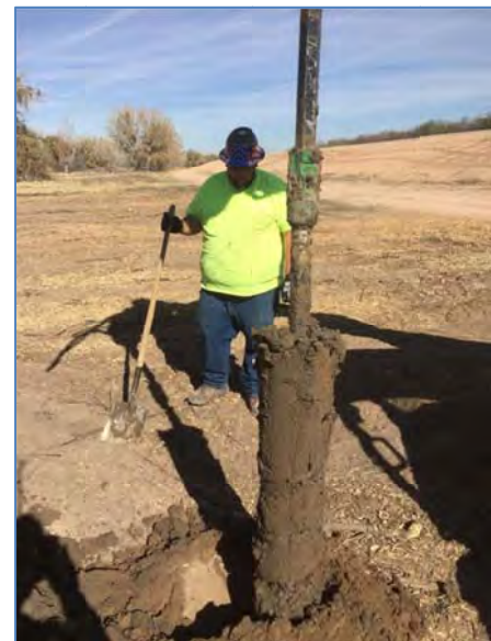
Augering holes for cottonwood pole planting at Sunland Park, 21 March 2018
