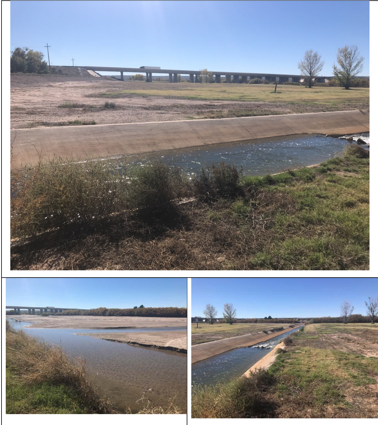
Figure 14. Representative field photos from the Las Cruces Effluent site. Top: Looking downstream across effluent discharge canal with adjacent eastside floodplain where constructed canal is proposed. Bottom left: Rio Grande downstream of the effluent canal. Bottom right: Effluent discharge canal flowing towards Rio Grande.
