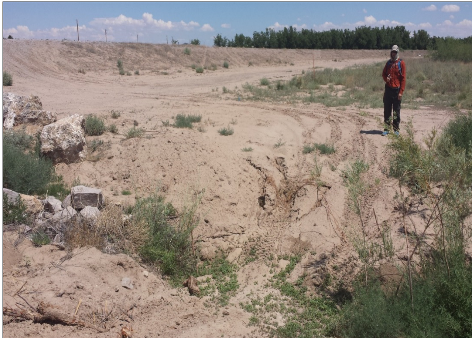
Figure 4.3. Off-road driving has continued over and through a constructed swale (Center Swale, Berino West).
