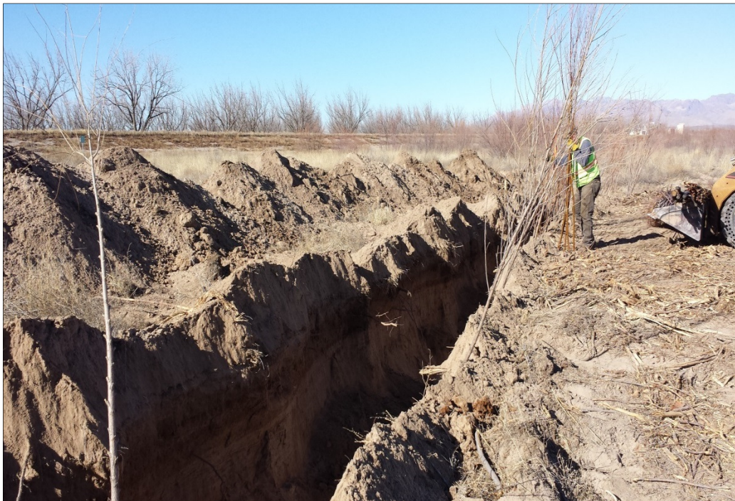
Figure 3.4. Planting willows into an excavated trench in a swale habitat (North Swale, Berino West).
