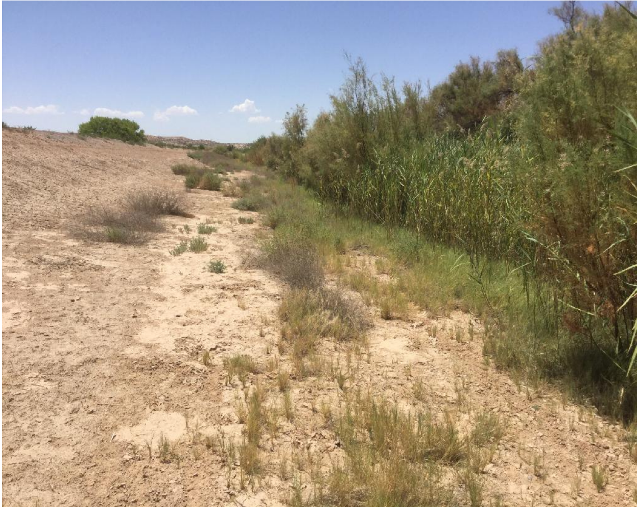
Photograph 2-7. MID levee toe, looking upstream (GSA 2021)
