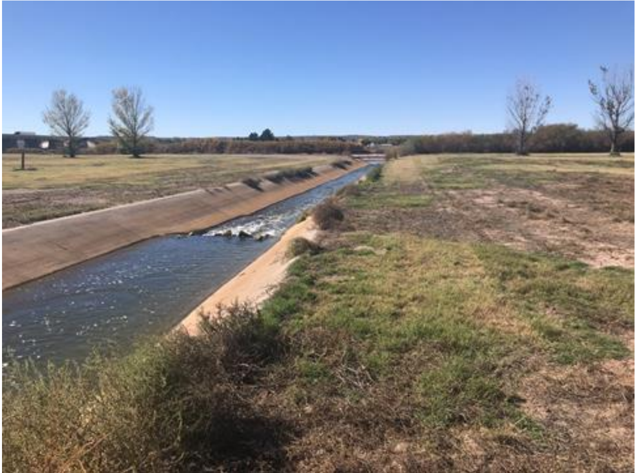
Photograph 2-3. Las Cruces concrete-lined effluent outfall channel
