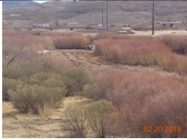
Contractors harvested willows from large islands in the river below Racetrack Drive, February 2018.
