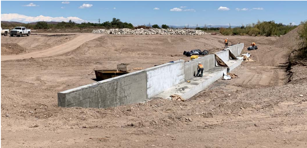
Figure 36 Construction of the endwall at Thurman I Arroyo Sediment Basin, March 2019
