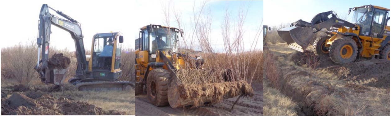
Figure 19 Transplanting island vegetation at Anapra Restoration site, January 2018. Left: Excavator creates trenches about 8 to 10 feet deep to groundwater; middle: a bucket of island willows with about 1 foot of topsoil; right: willows with roots are dropped into excavated trenches and backfilled.
