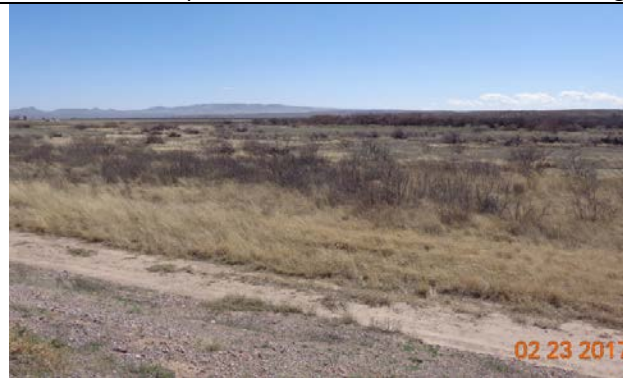
Contractor has started saltcedar removal, Feb 2017
