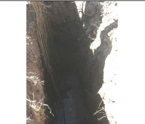
Depth to water during trenching in March 2016 shows favorable groundwater conditions
