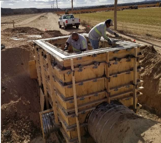
EBID constructing a box at Trujillo Lateral in Dec 2018
