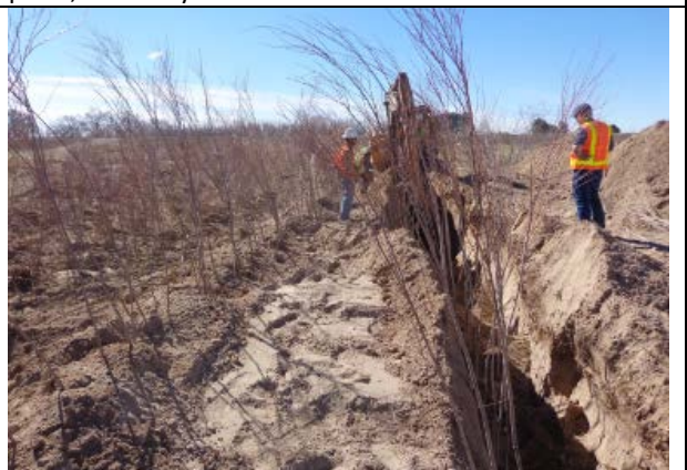
Contractors planted dense coyote willows in an old abandoned irrigation ditch via trench planting, February 2015 (left and right).
