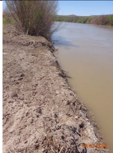
Monitoring water levels at another bank cut, April 2018.
