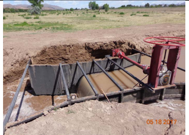
New turnout structure breached and irrigation had to stop. May 2017. Turnout was repaired by EBID in the following month.
