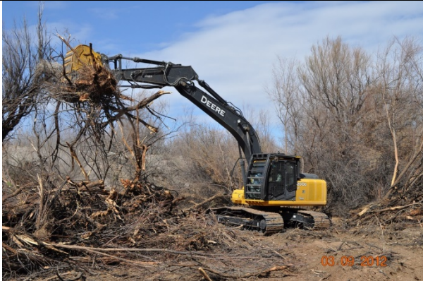
Monotypic saltcedar was removed with an excavator March 2012
