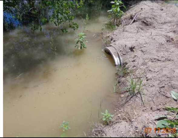
Water entering the second irrigation cell via the RCP, July 2018
