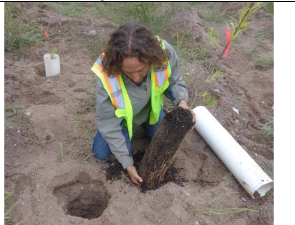
Subcontractor grew shrubs in extra tall pots in large PVC tubes and planted in augered holes. Sept 2017
