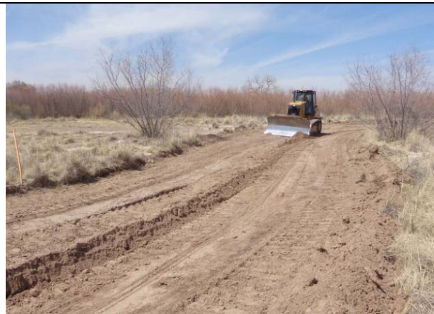
IDEALS begins excavation of swales at the site, March 2018.
