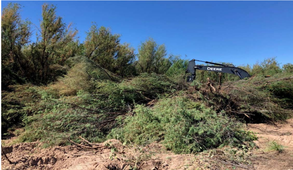
Figure 8 USFWS saltcedar removal at Rincon Siphon A site, September 2018
