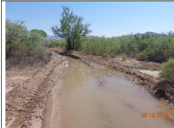
Successful water distribution channel constructed by USFWS, June 2019
