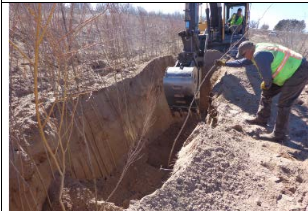
Contractors planted dense coyote willows in an old abandoned irrigation ditch via trench planting, February 2015 (left and right).
