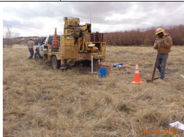
USIBWC well contractor EGC redrilling well at Country Club East, February 2018.
