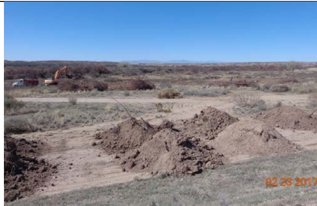
After saltcedar removal, contractors began excavating swales for planting, February 2017.
