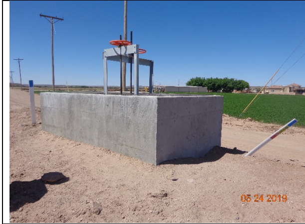
Completed turnout structure, May 2019
