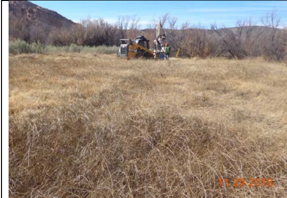
New monitoring well being drilled at northern boundary of site, Nov 2018.
