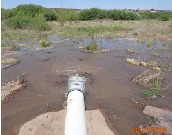
T-pipe connection to second irrigation cell, June 2018
