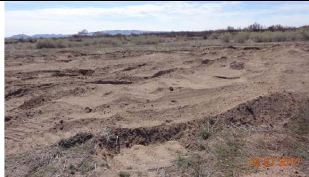
Excavated swale, February 2017
