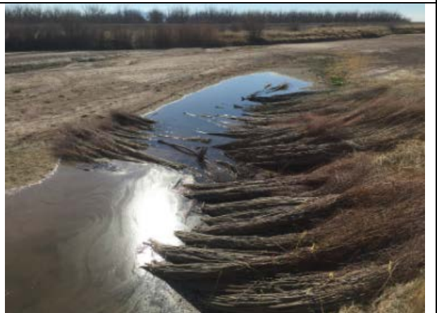
Willow poles were stored in the riverbed in a pond of water from the upstream Vado wastewater treatment plant, February 2015
