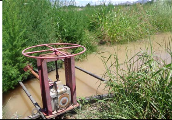
EBID turnout structure being closed after the irrigation is complete, July 2018.
