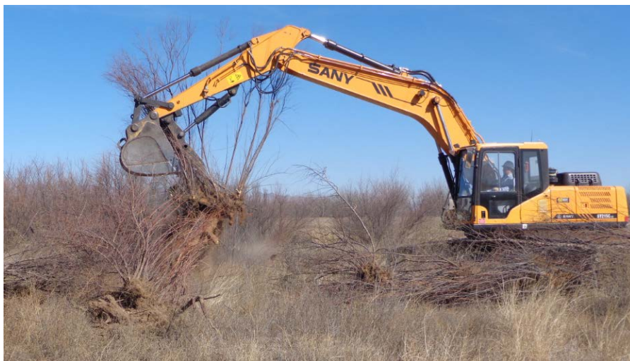
Figure 9 USIBWC contractors excavate saltcedar at Berino West Restoration Site, January 2015
