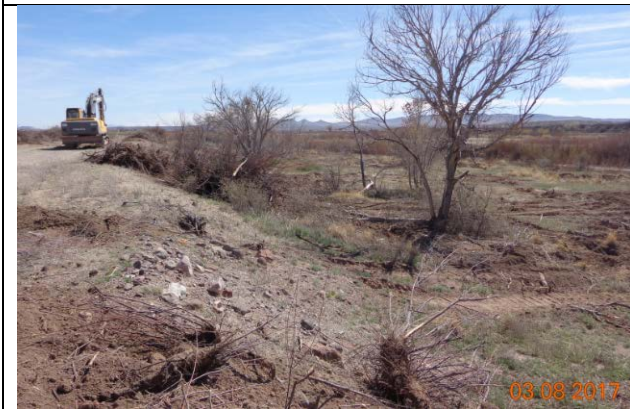
Saltcedar excavation at CCC, March 2017
