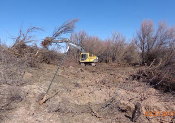
Saltcedar excavation February 2017
