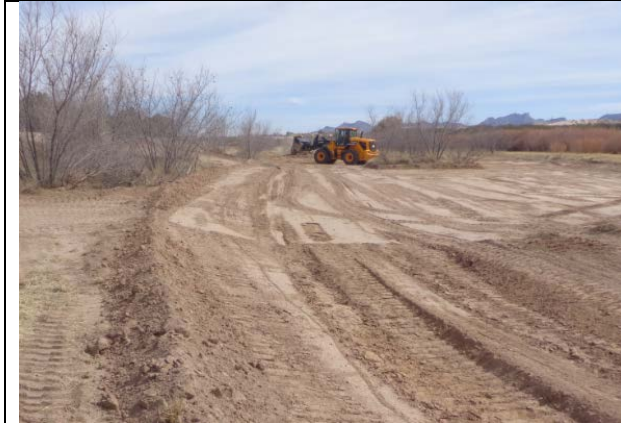
Excavation of large swales continues, March 2018.
