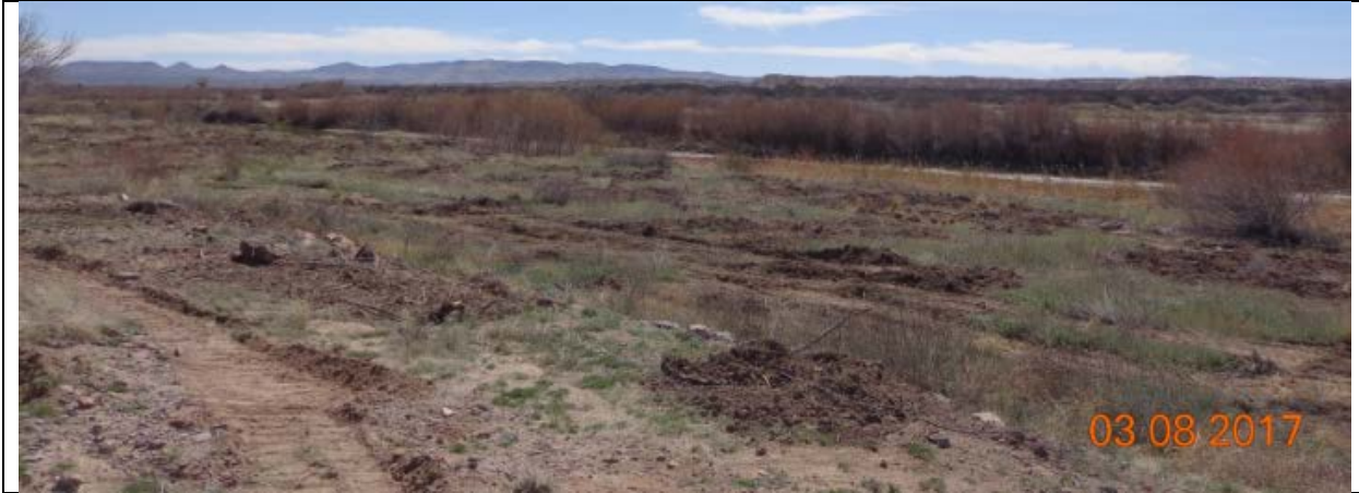
Site after saltcedar excavation, March 2017.
