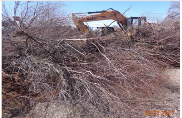
Saltcedar excavation February 2017
