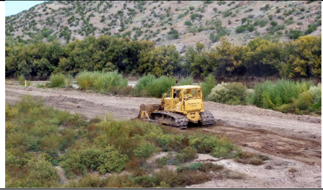
Lowering the floodplain to create a larger lower terrace to plant willows for flycatcher habitat, October 2014
