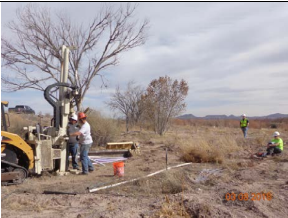
Groundwater monitoring well being redrilled using a track mounted geoprobe to limit disturbance to plantings. March 2018
