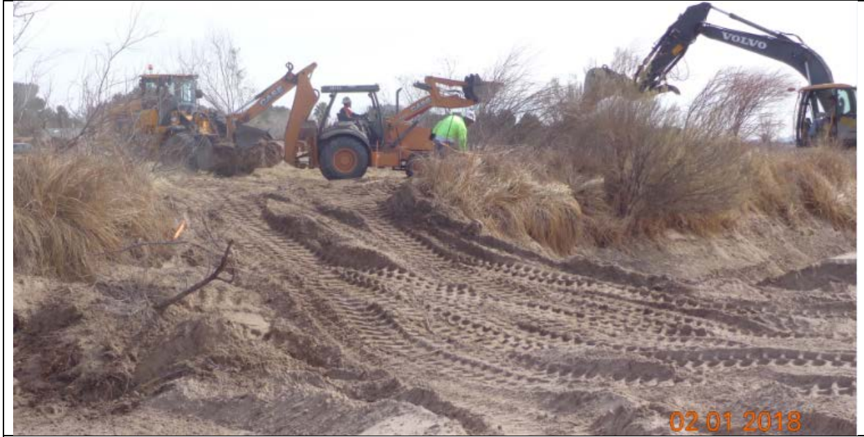
Heavy equipment crews transplanting harvested willows, February 2018.
