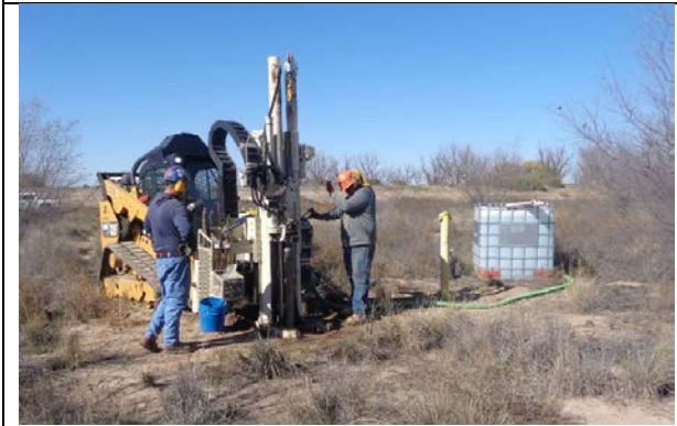
Drilling new well at Berino West, Nov 2018.
