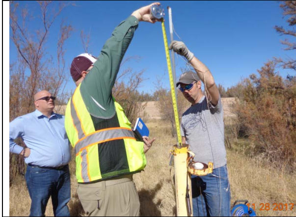
Contractors EGC conduct well assessment, November 2018.
