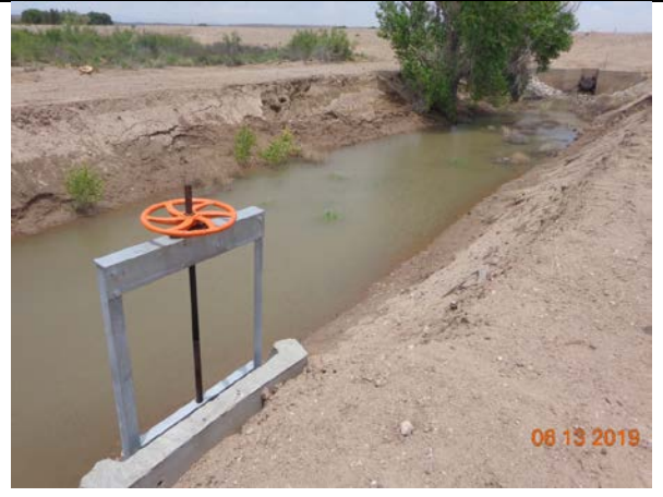
Check gate constructed by EBID on the Palmer Lateral used to irrigate the Yeso East site. June 2019
