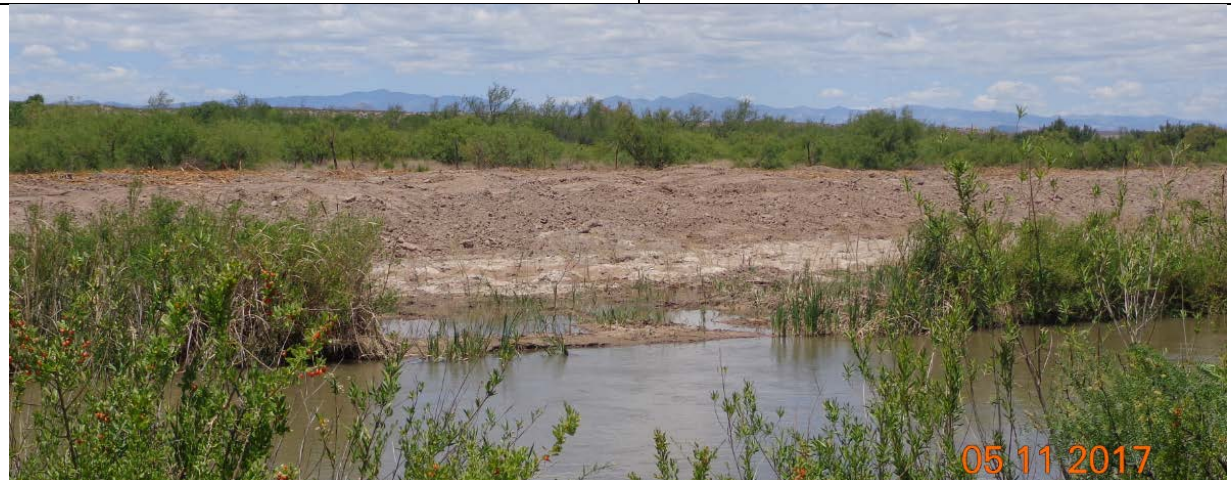
From Yeso East, looking towards Yeso West at the excavated inlet channel which is allowing some water to enter the site during normal flows at the beginning of irrigation season. May 2017
