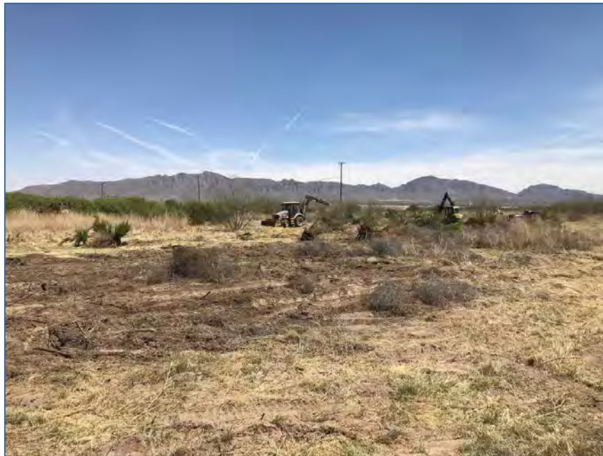
Saltcedar extraction at Vinton B, 24 April 2018
