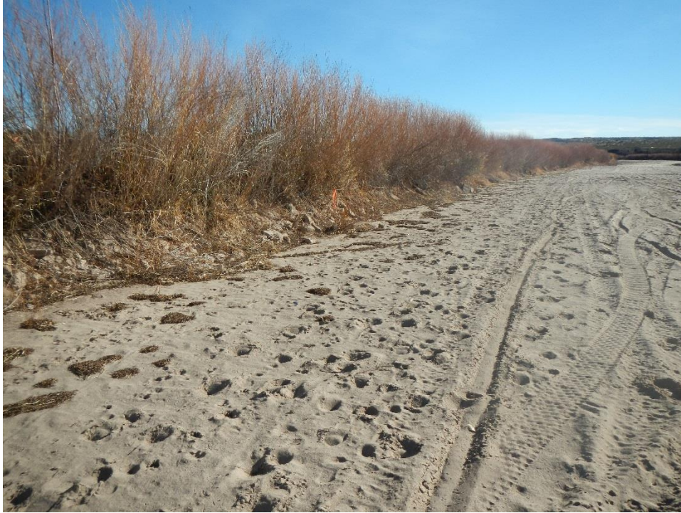
Photo A.77. View downstream to riprap bank protection along the left (east) bank in the vicinity of the Nemexas Siphon at the downstream limit of the Problem Location 8 reach.
