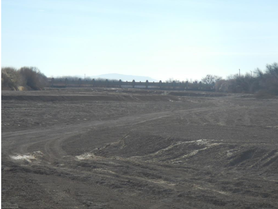
Photo A.61. View downstream to the depositional bars in the backwater zone upstream from Mesilla Dam.
