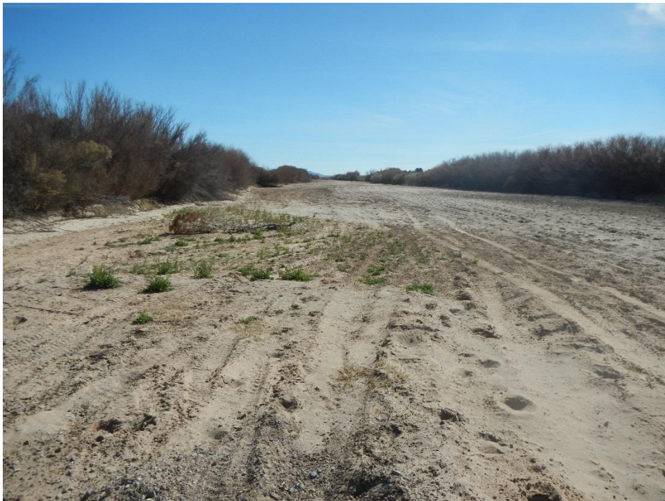
Photo A.71. View downstream from the mouth of the arroyo at Sta 806+50 where there is no alluvial fan, suggesting this tributary has not recently delivered significant sediment loading to the Problem Location 7 reach.
