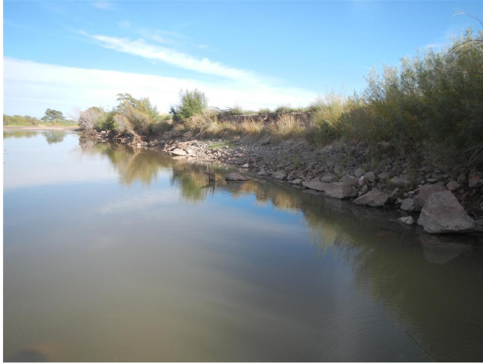
Photo A.21. View downstream along right bank of RGCP opposite the Thurman II Arroyo where coarse fan materials appear to have been placed to protect the bank.
