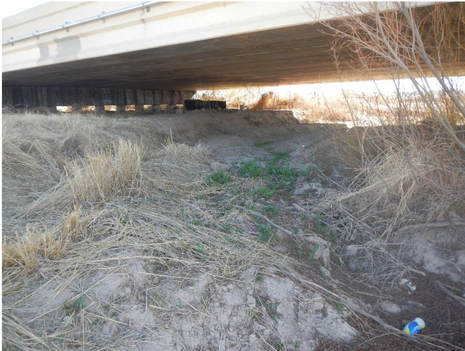
Photo A.73. View downstream to the eroding left bank under Country Club Bridge that is a result of flows deflecting off of the debris on Pier Set no. 2 (not shown in photograph).
