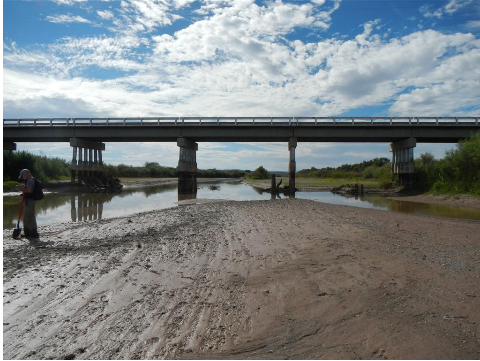
Photo A.15. View upstream to the Salem Bridge (New Mexico Highway 391).
