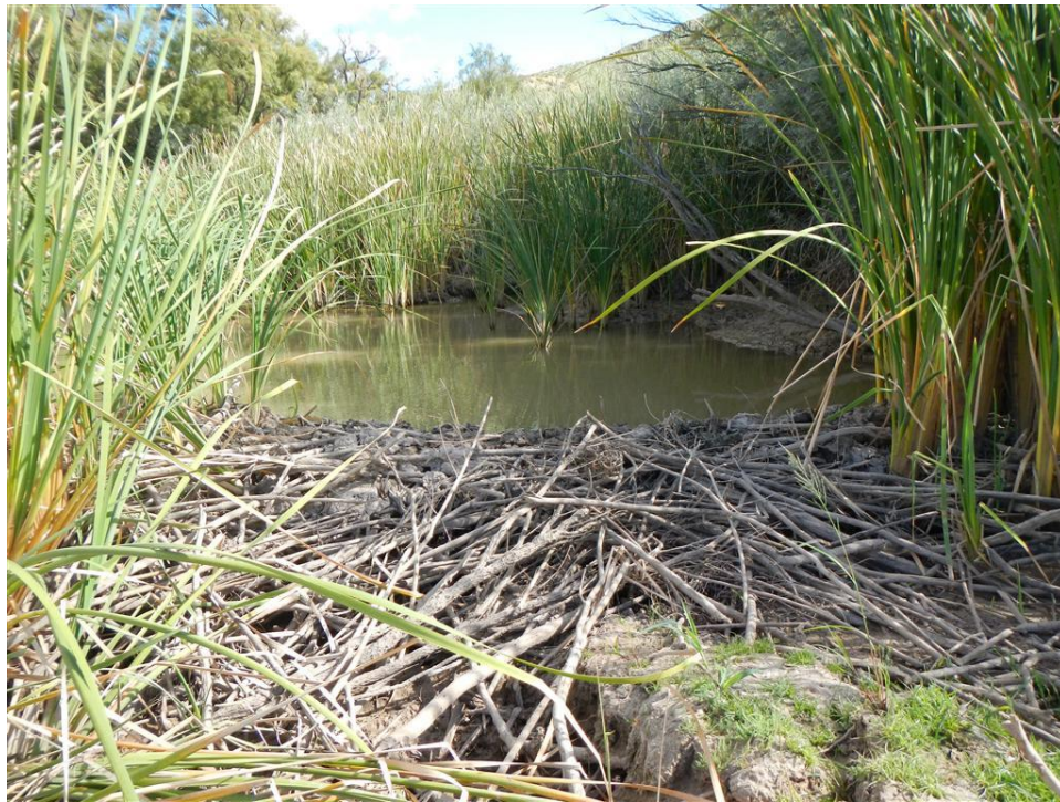
Photo A.50. View to outlet of Rincon/Tonuco Drain that is affected by beaver activities.
