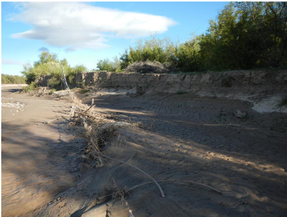
Photo A.46. View looking upstream along the eroding east bank of the river opposite the Rock Canyon fan.
