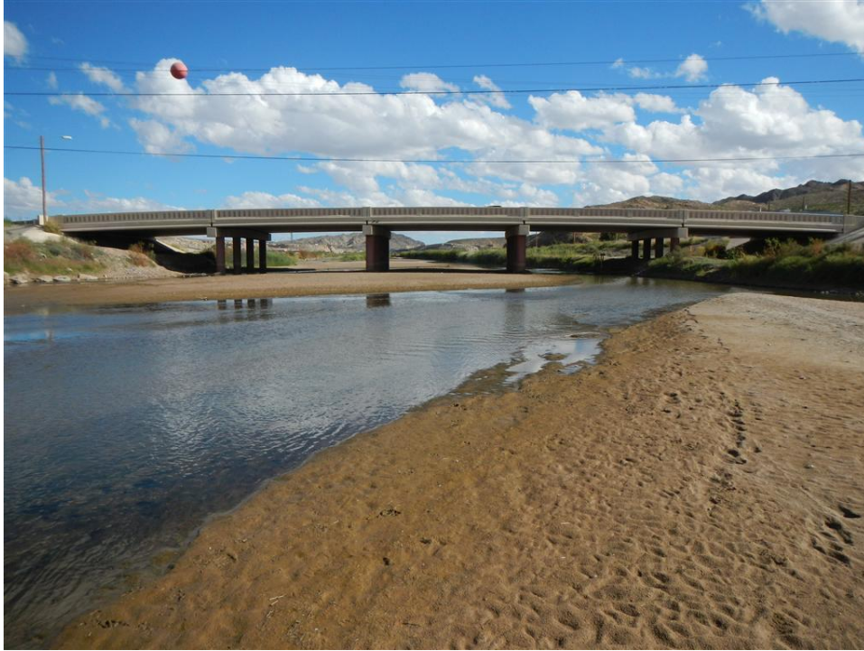
Photo A.79. View downstream to Courchesne Bridge (McNutt Road).
