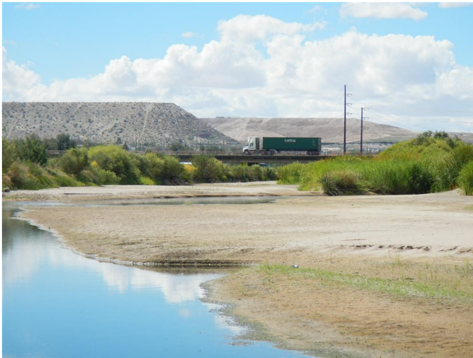
Photo A.78. View upstream to Anapra Bridge (Racetrack Drive).
