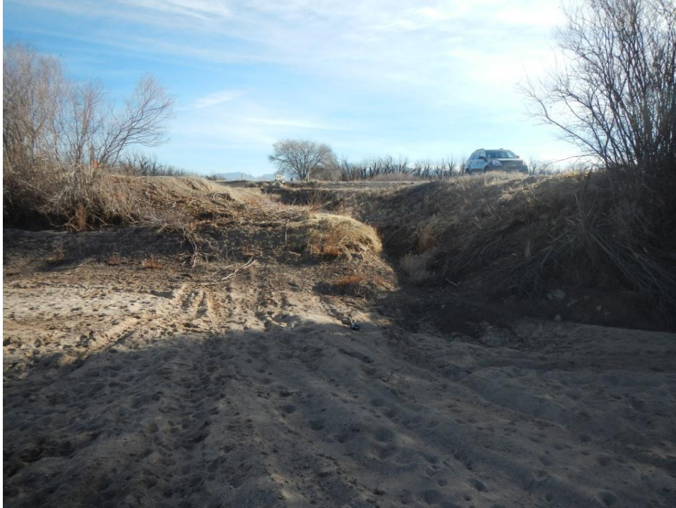
Photo A.55. View of the mouth of drain for the California Lateral, where the invert of the drain is at approximately the same elevation as the riverbed.
