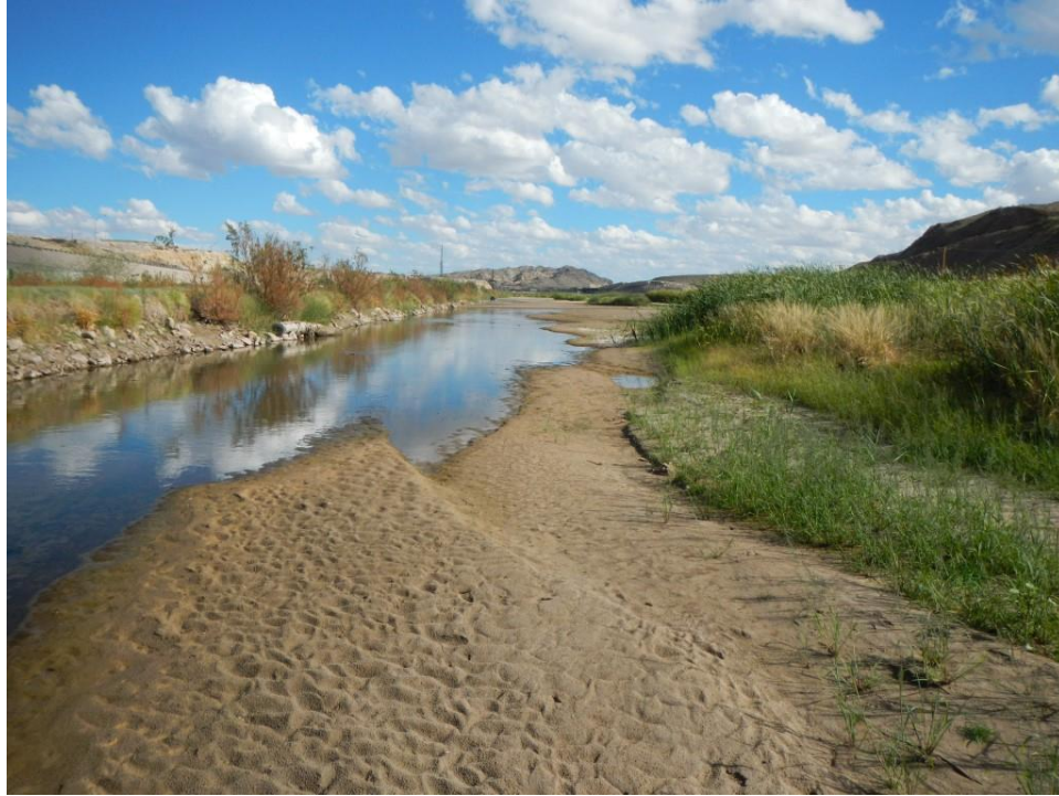
Photo A.87. View downstream along the left bank downstream from the Courchesne Bridge (McNutt Road) where riprap bank protection is visible.
