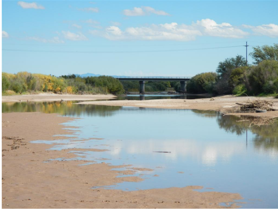
Photo A.33. View downstream to the New Mexico Highway 140 Bridge near the upstream limit of the Problem Location 4 reach.
