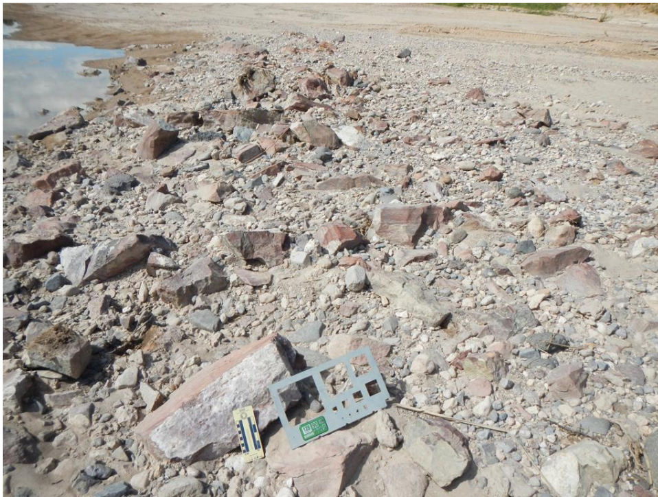
Photo A.35. View upstream along the west bank opposite the Rincon Arroyo fan, where fan materials have been placed along the toe of the bank but erosion of the upper bank has continued.
