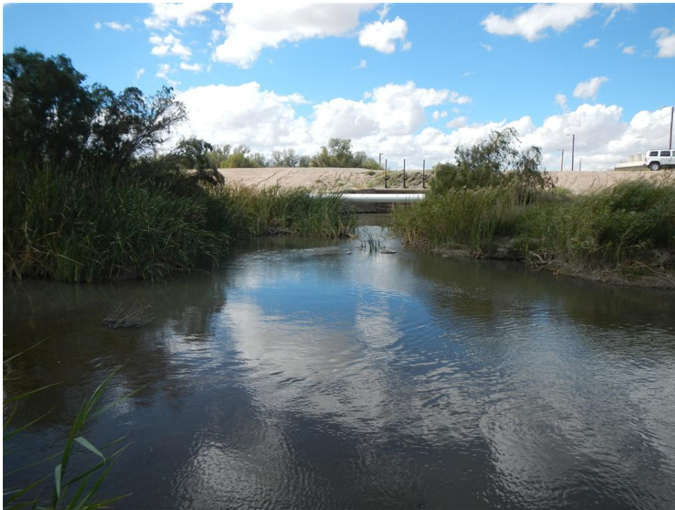
Photo A.86. View across left side channel to the Montoya Drain outlet.
