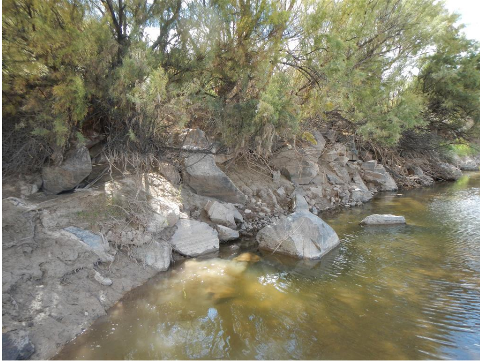
Photo A.51. View downstream to the riprap-protected east bank downstream from the Rincon/Tonuco Drain.
