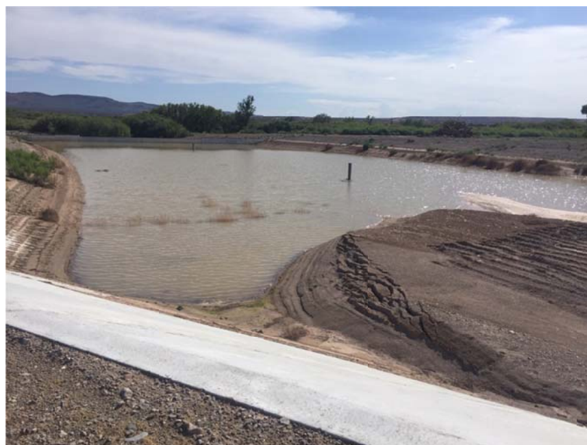
Sediment basin after construction at Thurman II Arroyo (28 August 2019).
