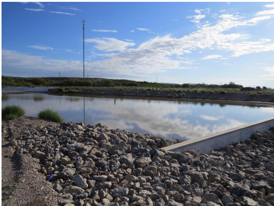
Sediment basin after construction at Thurman I Arroyo (14 October 2019).
