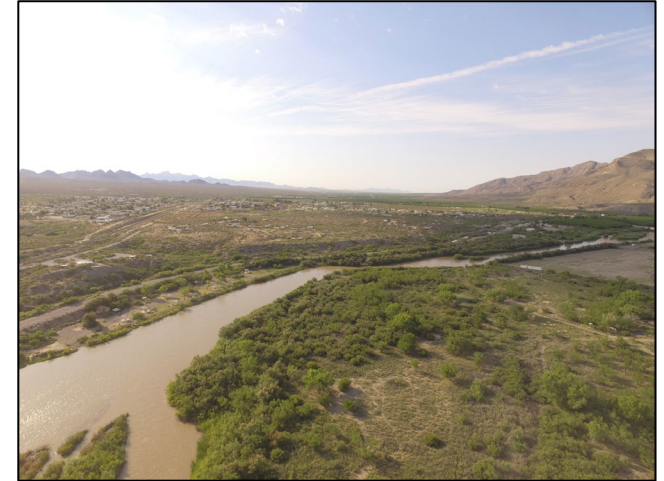
Potential off-channel site at Leasburg Diversion Dam, courtesy of EBID
