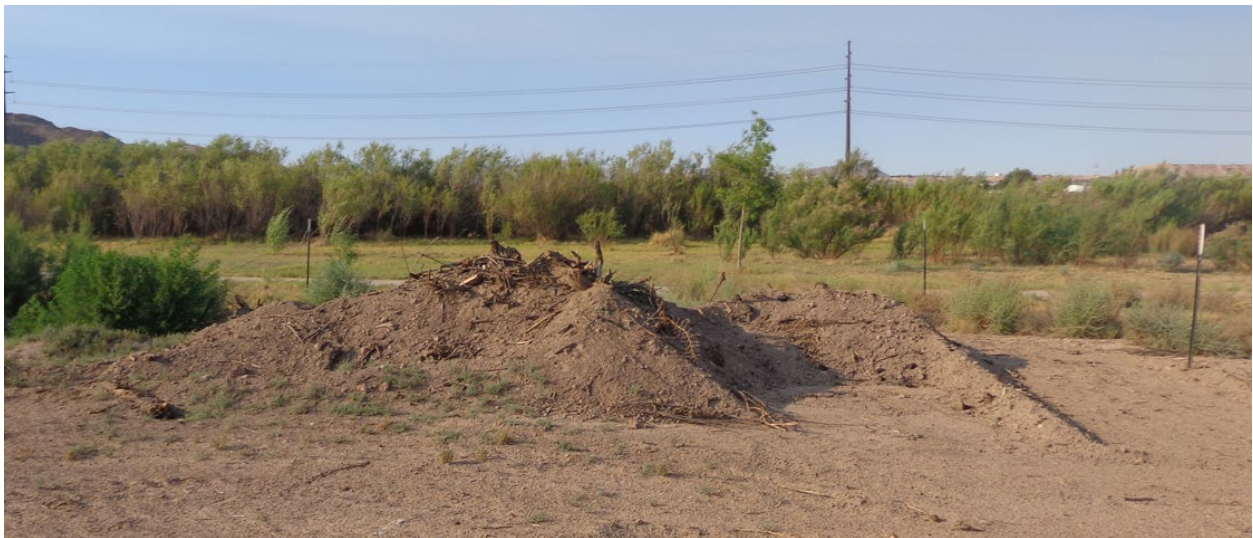
A sediment pile is still remaining.
