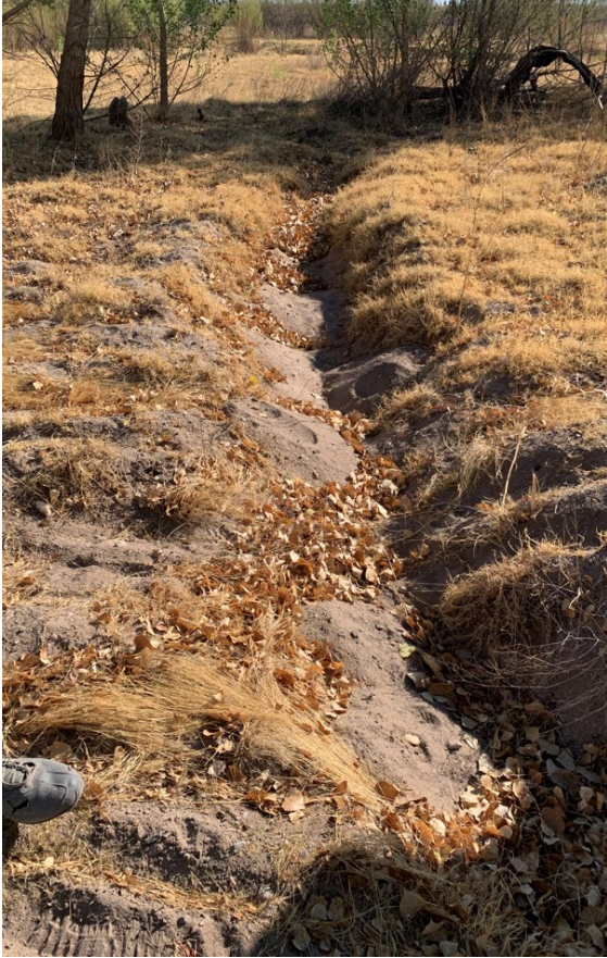
Earthen v-ditch to convey irrigation water around the site (dry, left, and full, right).
