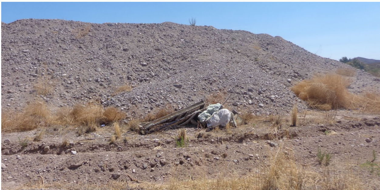
Spoil pile in the northern end of the site is about 30 feet high. This portion of the site is unrestorable and should be excluded from the site. The EA considered excavating this as part of the arroyo terracing, but costs and logistics to remove such a pile is cost prohibitive.
