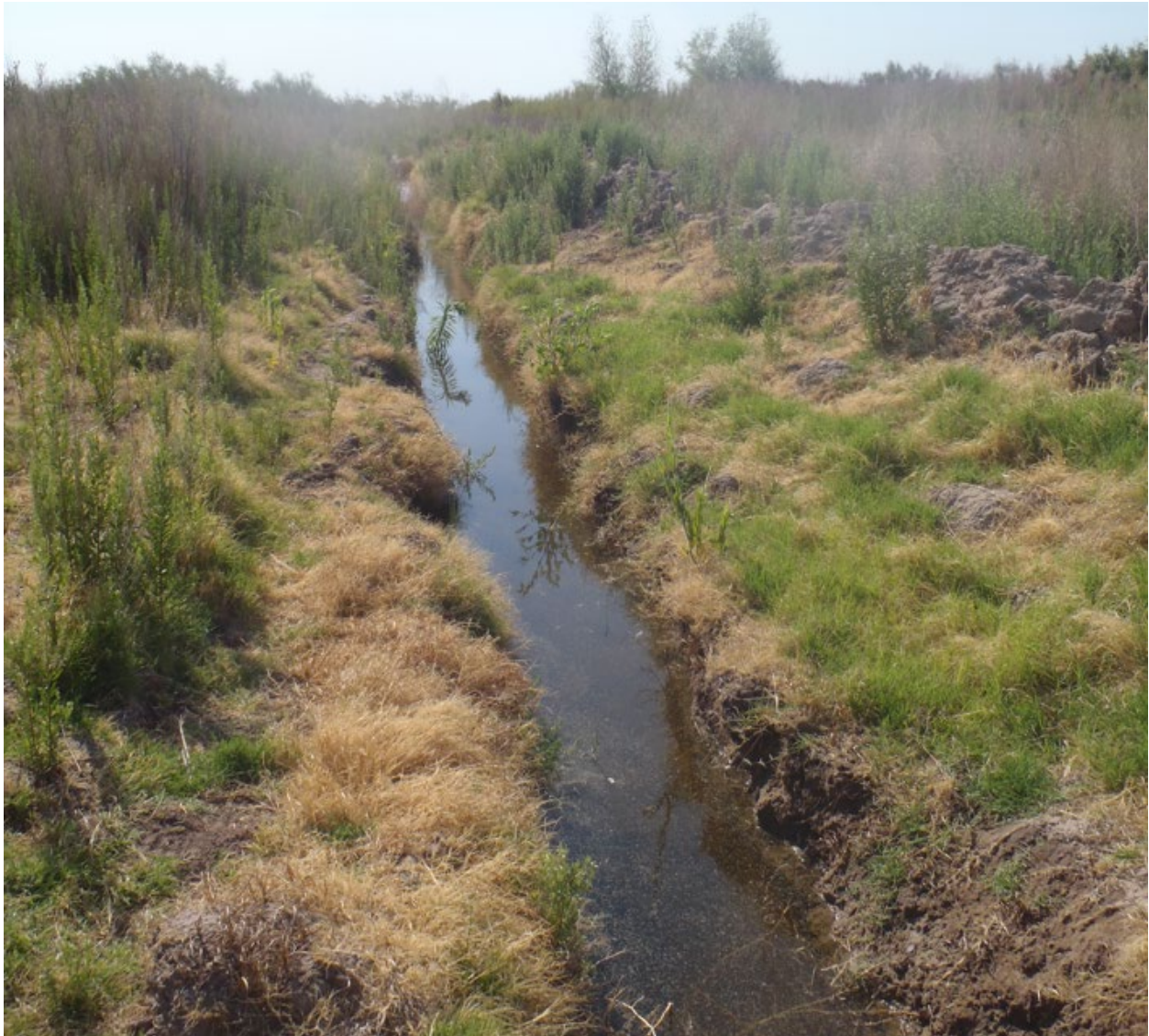
Earthen v-ditch conveying irrigation water from Garfield Canal upstream through the site.
